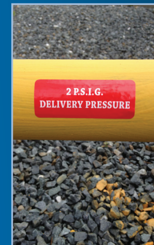
Sample of piping label used to identify elevated delivery pressure piping.
